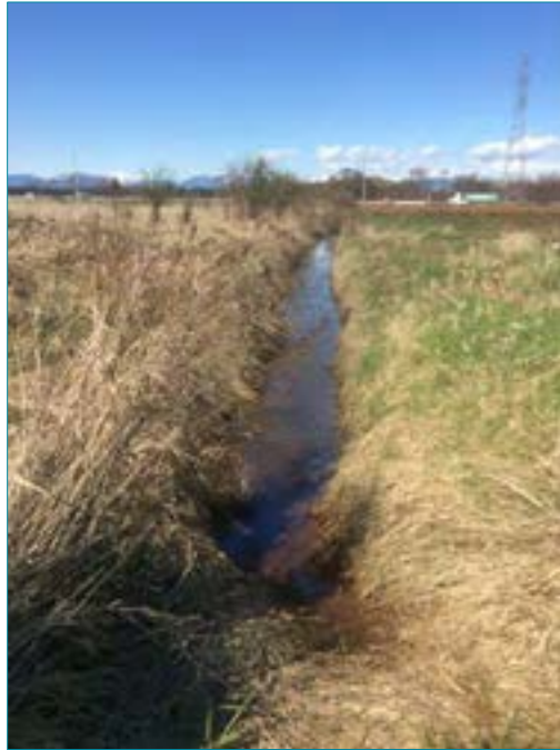
Photo 76: Representative photo of Delta Agricultural Ditch #11 99 (Watercourse #78), looking north from Ladner Trunk Road. April 1, 2014.
