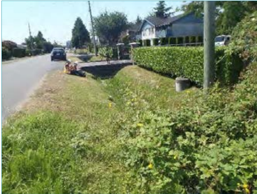
Photo 3: Representative photo of Patterson Road Ditch North (Watercourse #8), facing west. July 14, 2014.
