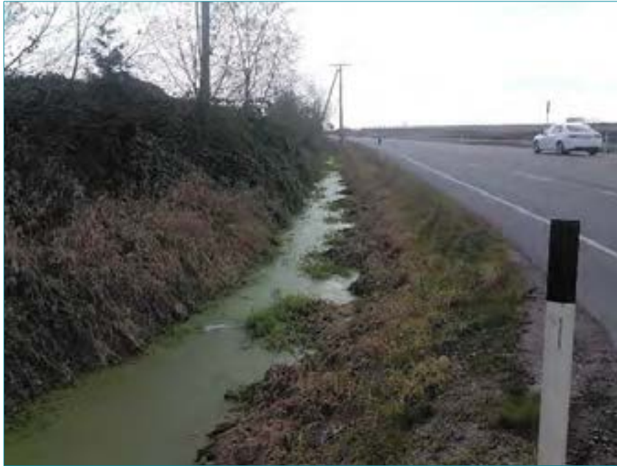
Photo 78: Representative photo of 80 street Ditch East, south of Highway 99 (Watercourse #80), looking south from Ladner Trunk Road. October 17, 2014.
