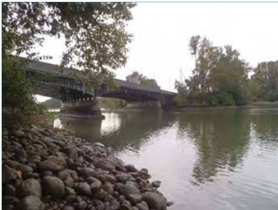
Photo 48: Deas Slough (Watercourse #51), facing downstream from south bank at Highway 99. February 19, 2014.
