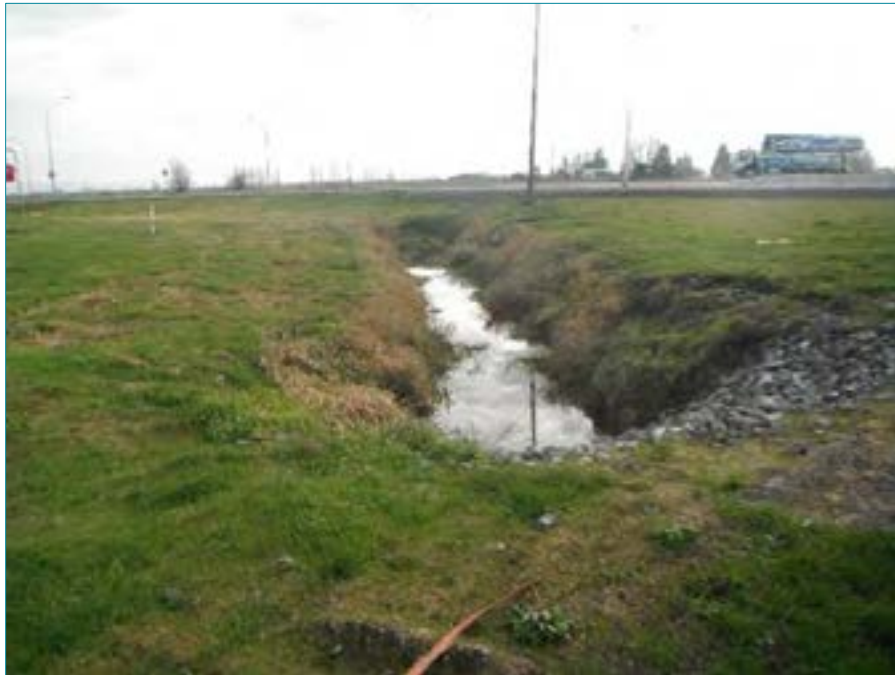
Photo 95: View of Ladner Trunk Road Interchange Northeast Outer Ditch (Watercourse #99), facing southwest. October 18, 2014.
