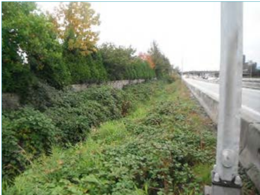
Photo 6: Representative photo of Highway 99 Ditch West (between Cambie & Shell) (Watercourse #11), facing northwest. October 17, 2014.
