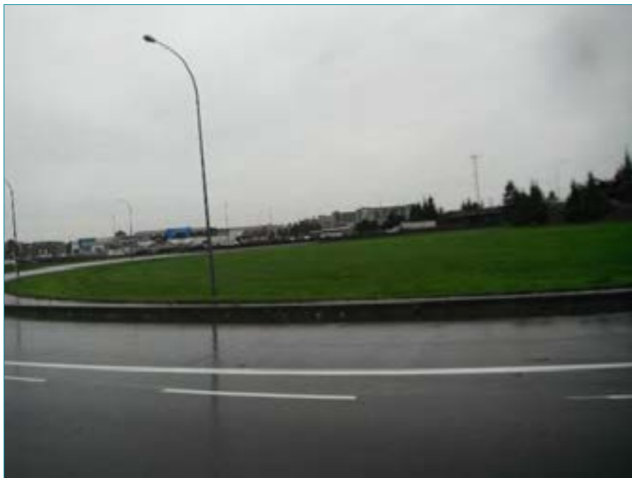
Photo 36: View of Steveston Highway Interchange Southeast Ditch (Watercourse #42), facing west. October 17, 2014.
