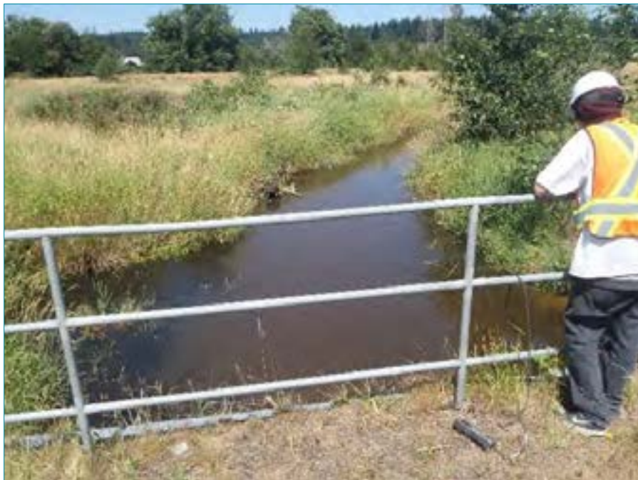
Photo 110: Representative photo of Eugene Creek Diversion (Watercourse #115), facing north. July 15, 2014.
