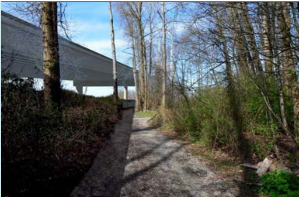
Figure 20 Simulated Future Viewscape from Viewpoint 9 (Millennium Trail between River Woods Neighbourhood and Highway 99)
