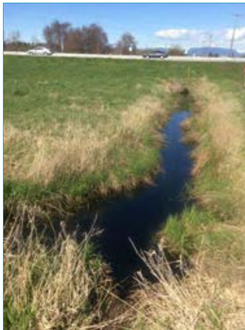
Photo 85: Representative photo of 88 Street Ditch West, south of Highway 99 (Watercourse #89). Taken from Ladner Trunk Road looking north. April 1, 2014.
