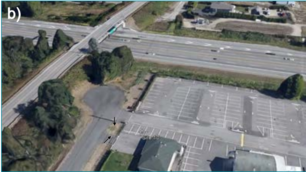
Figure 17 a) Photo of Microphone Site, and b) Aerial View of Noise Sampling Site October 31 - November 1, 2013 (Noise Levels in 15 minute Intervals)
