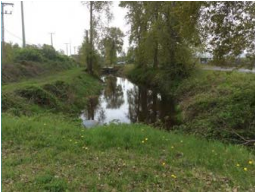
Photo 38: Representative photo of Highway 99 Ditch West (between Steveston and Fraser River) (Watercourse #44), facing south from Rice Mill Road. April 21, 2014.
