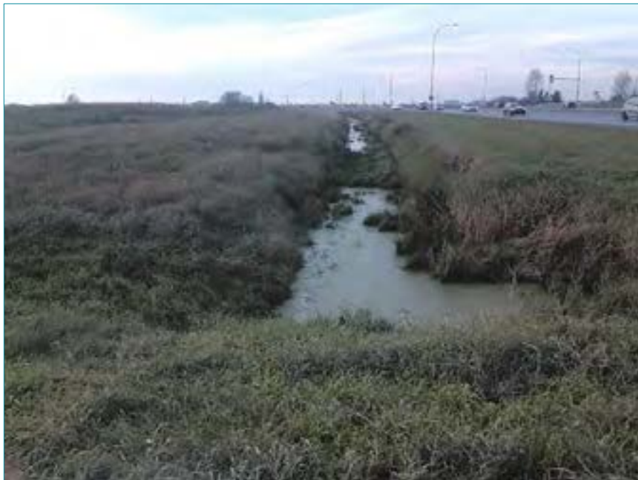
Photo 108: Representative photo of Highway 91 Interchange South Outer Ditch (Watercourse #113), facing west from Highway 91 overpass. October 17, 2014.
