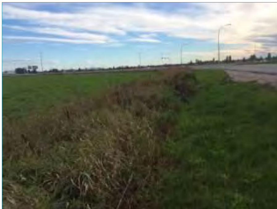
Photo 56: Looking southeast at Highway 99 Ditch Northeast (between 17A and 64 St) (Watercourse #57) from River Road exit. October 19, 2014.
