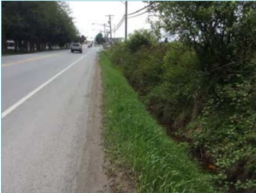
Photo 33: Representative photo of Steveston Highway Ditch North, east of Highway 99 (Watercourse #39), facing west. April 21, 2014.
