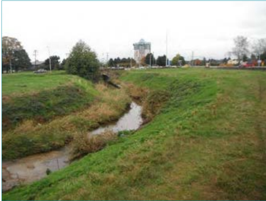
Photo 5: Representative photo of Tuttle Avenue Ditch East (Watercourse #10), facing downstream. October 17, 2014.
